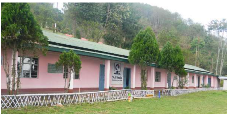
IGNOU Centre & Skill Development Centre
